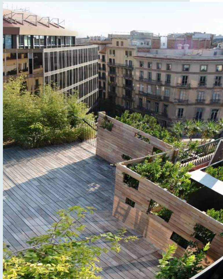
Wooden decking and wooden walls with framed views characterize the roof garden of "La Casa por el Tejado" providing a special meeting place for the employees of "La Casa por el Tejado". © Ira Irina Ivanova
