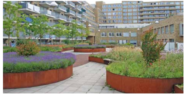
Courtyard C – an ecological interpretation of butterfly wings. © ZinCo Benelux, Harmen Riemens
