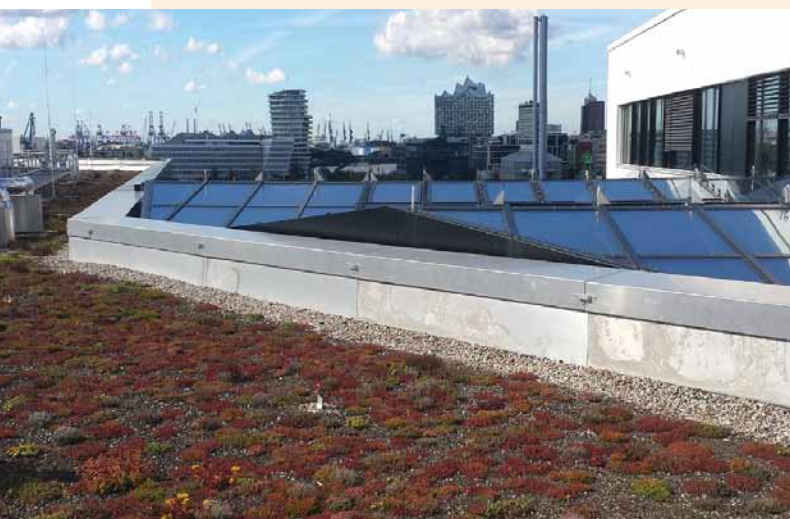
View over the HCU extensive Green Roof. © Hafencity University Hamburg
