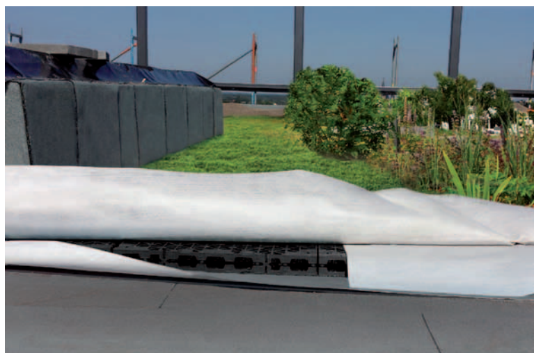
The spacer creates space to store the water, while above it virtually any type of Green Roof and roof utilisation is possible. © Zinco GmbH
