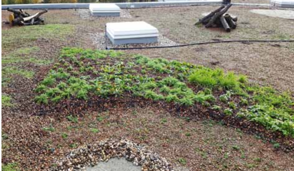
A mixture of herbs and grasses was planted on the substrate mounds in September 2016. © DDV
