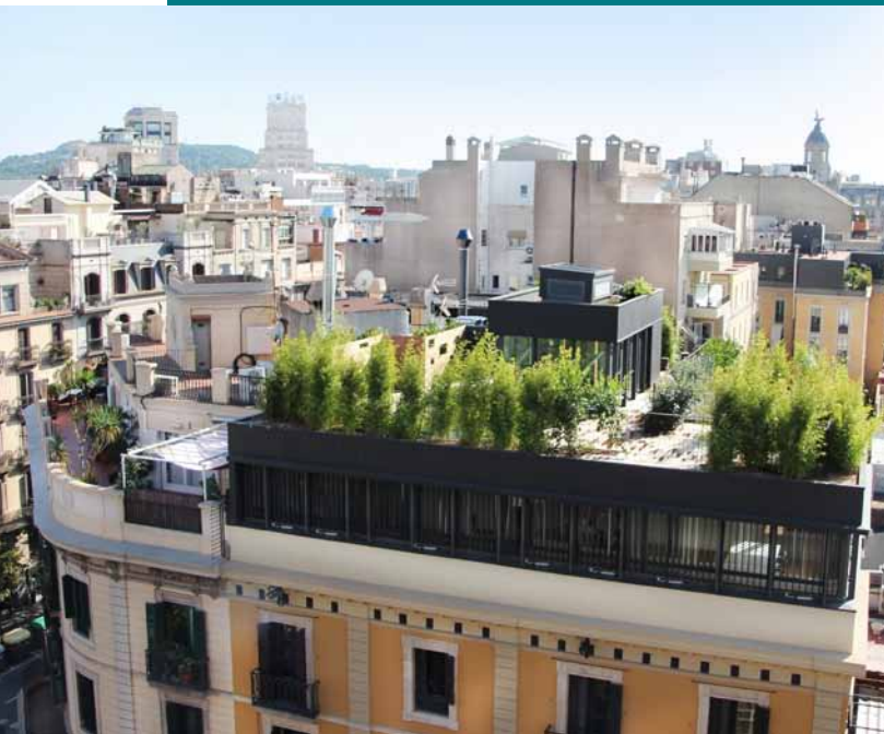
A bird's eye view of the head office roof garden of “La Casa por el Tejado” in the district of Eixample in Barcelona. © Ira Irina Ivanova
