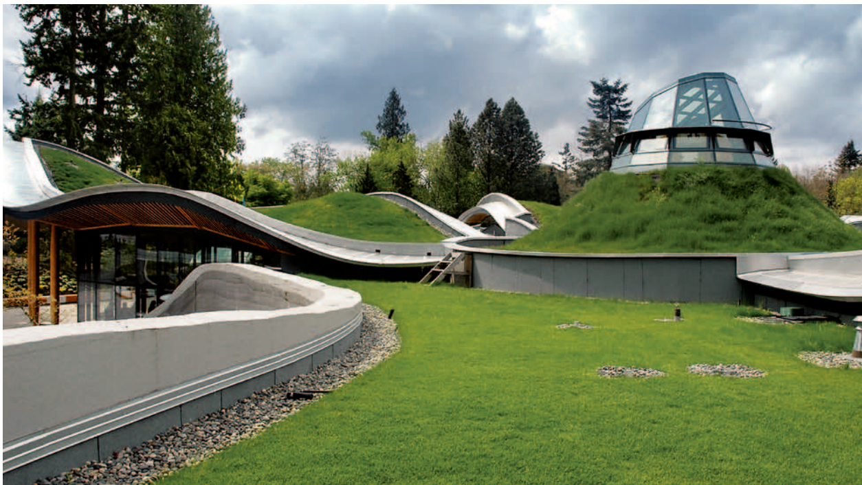
An outstanding example for sustainable stormwater management with Green Roofs – The VanDusen Botanical Garden Visitor Centre in Vancouver, Canada. © ZinCo
